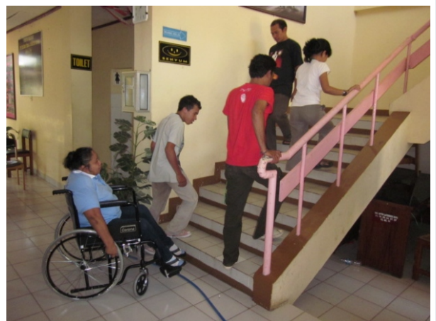
This picture taken during Mainstreaming Disability Issues in DRR Training in Kupang, displays an official building that is inaccessible to the persons with disabilities
